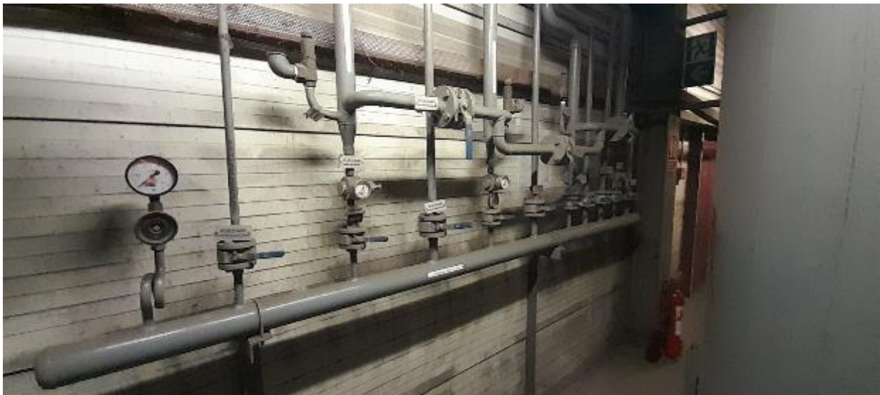
Fig. Connecting point of the nitrogen piping on E1A boiler house.
