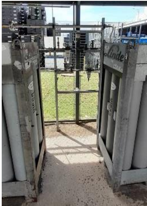
Fig. Connecting point of the nitrogen piping on E1A boiler house.
